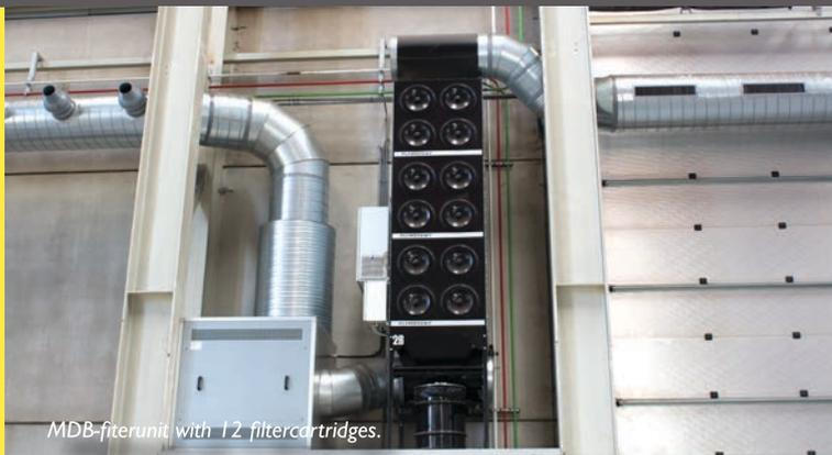
MDB-filterunit with 12 filtercartridges.
