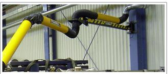
The FlexMax can be mounted in areas with a low ceiling (min. mounting height 2 m / 6.6 ft)
