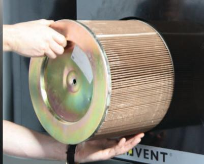
Filter replacement (CART filter) of the MultiDust® Bank
