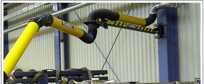
The FlexMax can be mounted in areas with a low ceiling (min. mounting height 2 m / 6.6 ft)
